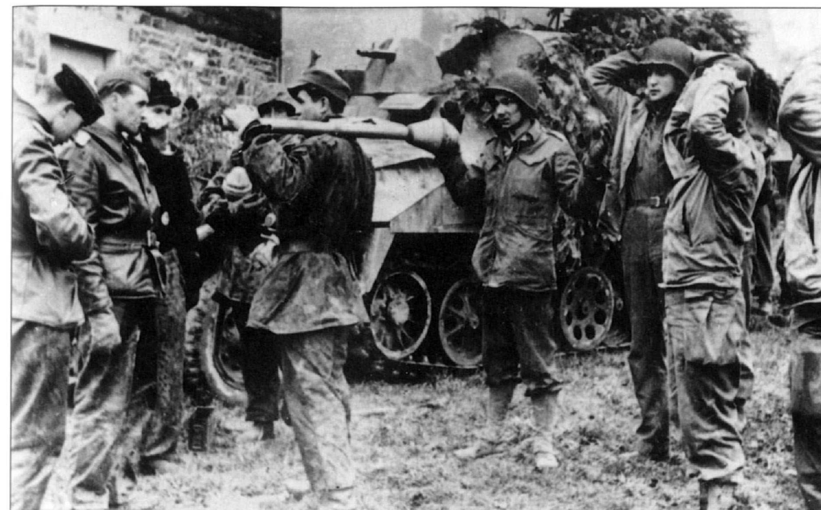
Left: A Sturmgeschütz (assault gun) or StuG of Sixth SS Panzer Army with accompanying SdKfz 251 half track. Assault guns, essentially tanks with no turret and a fixed gun, were cheaper and quicker to manufacture.
