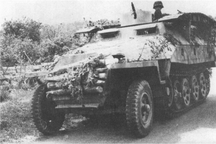
Schutzenpanzerwagen 251/7, a vehicle of the engineer troops, with crossing rails fastened to the side. Note the blackout headlight on left fender and the divisional insignia next to co-driver's hatch.
