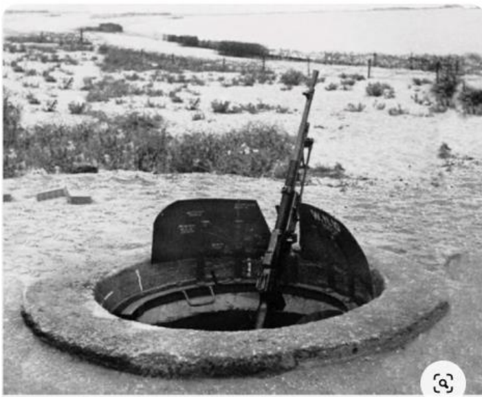
Tobrukstände with armour plate protection – note the range markings painted on the shield. The machine gun is a Czech LMG and the ancestor to the British Bren.
