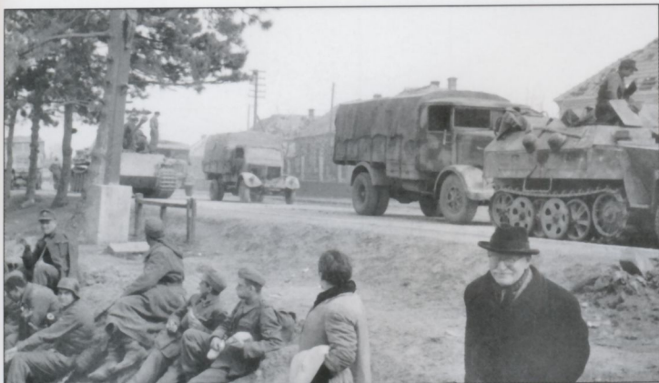
A column of transport trucks pass a Panther Ausf.G and an Sd.Kfz.250 'Neue' in a Hungarian town in March 1945 on their way to Lake Balaton, known as the Plattensee to the Germans. To help conceal the movement of 6.Panzer-Armee to the eastern front for the planned Operation 'Spring Awakening', all troops were ordered to remove their cuffbands, as evidenced in this photo and all units were given special codenames. By 10 February 1945 the division had been brought almost back up to strength with 38 Pz.Kpfw.IV, 44 Panthers, 21 Jagdpanzer IV and 165 SPW's. (M. Bayerl)
