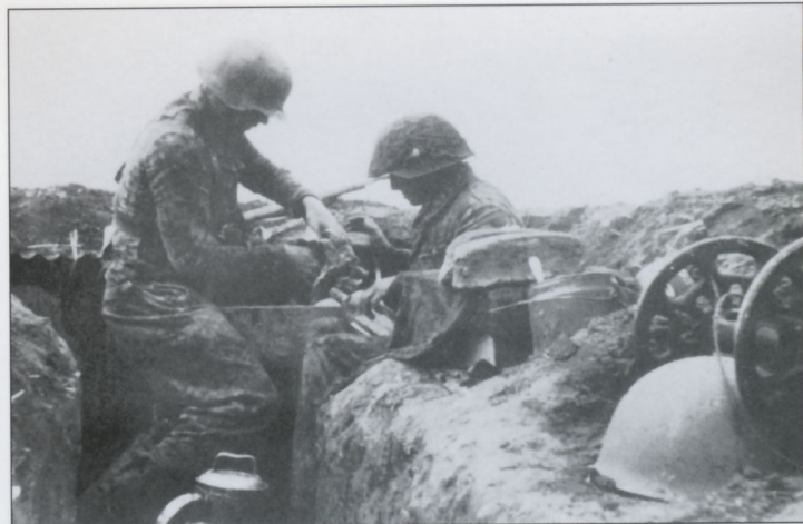
Two grenadiers from I./SS-Panzer-Grenadier-Regiment 25 take a meal break north of Caen in July 1944. Their elaborate dugout has a corrugated sheet metal roof reinforced with wood framing and covered with soil for protection. Two loaves of bread and their mess kits can be seen in the foreground along with a telephone cable reel.
